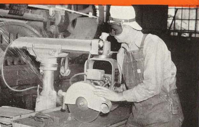
(Above) "Kick" cutting with a W-T Radial Cut-off machine.
