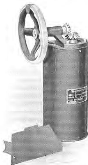
Four Speed Controller Top Cover removed to show Unit Assembly with Gears and Hand Wheel
