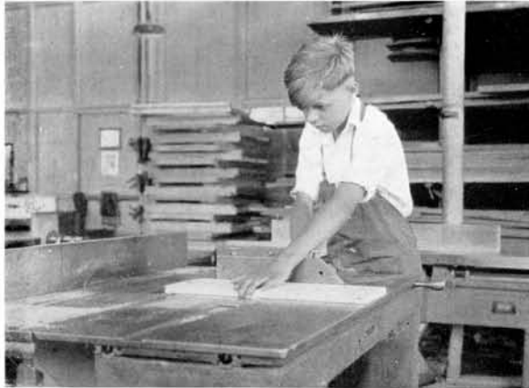
FIG. 26 Simple crosscutting— squaring first end
