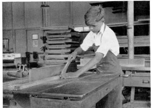
FIG. 21 Ripping narrow stock—use of push stick
