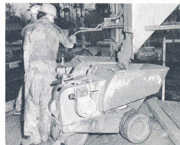
7-hp BKN on concrete buggy
