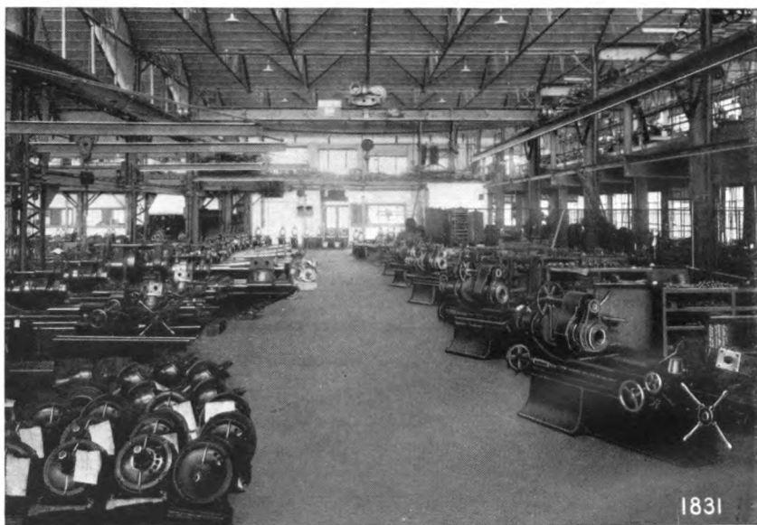
Interior View—Main Works
