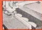
Layout marks are always in plain view on "top" of the board and easy to follow.
