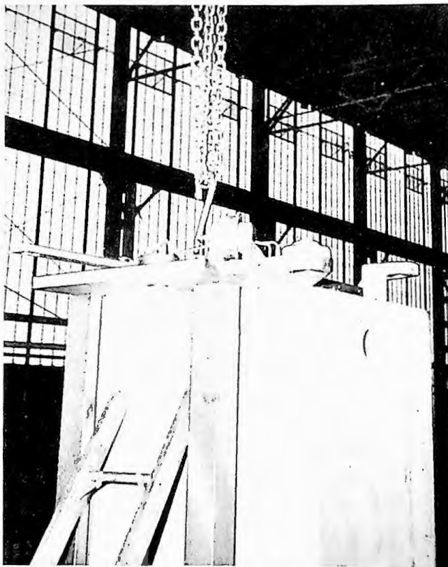
Figure 6. Mounting Sheave Bracket on Column
