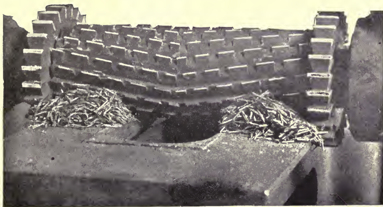
MILLING FACE AND SIDES AT ONE CUT.
