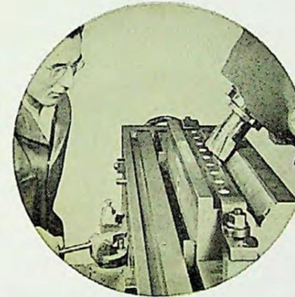
Angular milling • Here a V is being milled. Note that only the position of the cutterhead has been changed; workpiece is still in original position.
