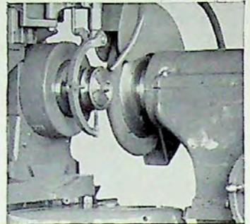
External grinding of inner race.
