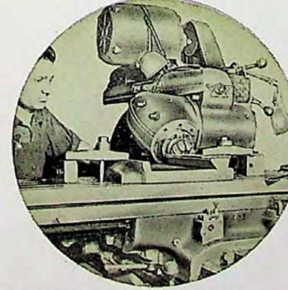
With head locked in angular position the operator is taking an angular cut and operates the miller with the rear directional controls.
