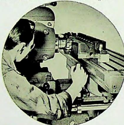
Horizontal milling • With adjustable cutterhead locked in horizontal position and the work set up, the operator uses rear controls and starts the job with a face milling operation.
