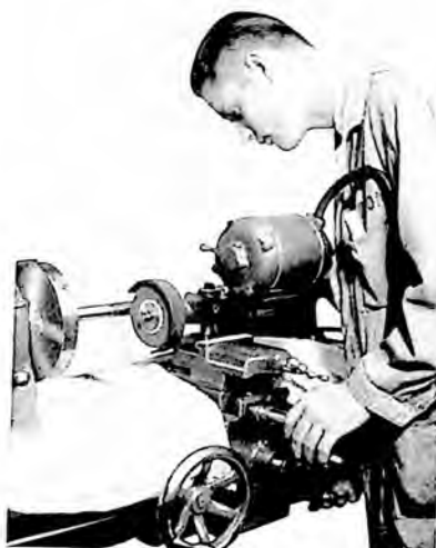
Grinding a Mandrel
