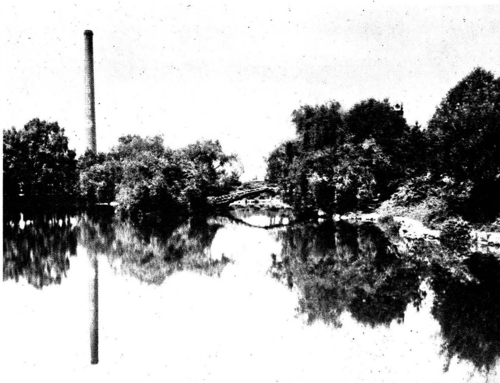
Power House Across Lake
