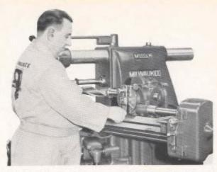
The Majority of Operators are Righthanded—That is why K&T have placed their dividing head at the right hand end of the table, to enable the operator to stand at his normal position ahead of the index crank, to index easily and naturally with his right hand and more accurately, too.
