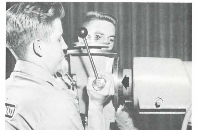
FIGURE 15B Removing Spindle Housing
