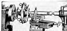
Truing Hub Flanges of Front or Rear Wheels
