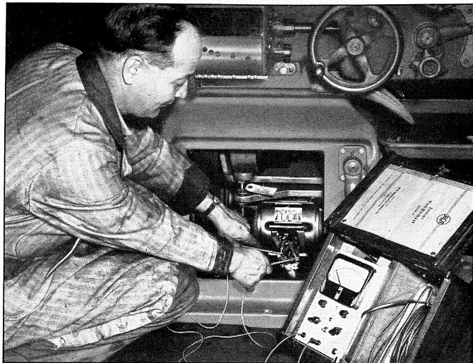
Fig. 2. Checking the line voltage at the motor.
