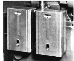
Line-starter Control Equipment for two-speed motor
