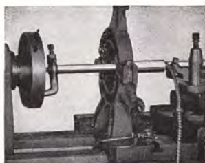
Fig. 88. Turning Long Work in the Center Rest.
