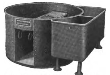
FIG. 12. STATIONARY DOWN DRAFT FORGE NO. D85-D
