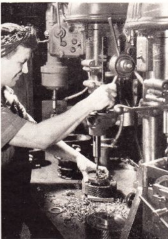
Drilling two \frac{5}{16} " diameter holes with high speed drill for \frac{3}{8} " tap in timing gear. Heat treated alloy steel Rockwell 40-42 C scale hardness. Slow speed attachment at 200 R.P.M.
