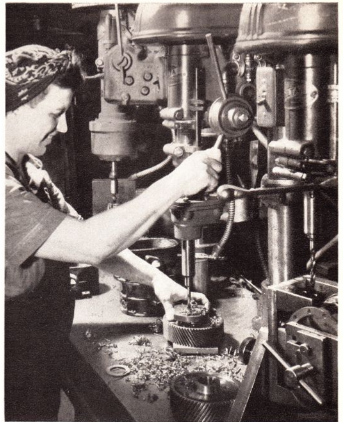
Drilling two \frac{5}{16} " diameter holes with high speed drill for \frac{3}{8} " tap in timing Gear. Heat treated alloy steel Rockwell 40-42 C scale hardness. Slow speed attachment at 200 R.P.M.
