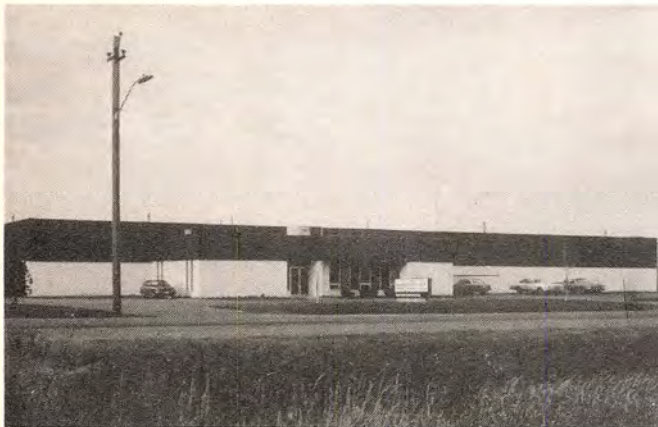
Canadian Distribution/Service Center, Guelph, Ontario, Canada
