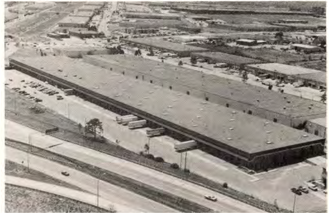
Distribution/Service Center, Memphis, TN
