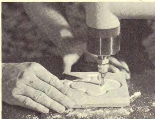
Routing using a guide pin and template.
