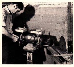
The standard tool grinder and the disk finishing machine . . . a perfect team for grinding, deburring, polishing.
