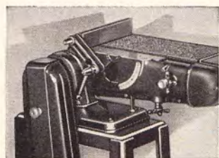
Above. View from rear, showing adjustable back stop and its bracket. This is available for use in sanding flat work, to prevent it from being carried along with the belt.
