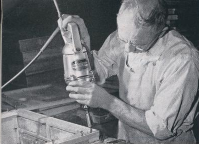
↑ Assembling heavy wooden cash drawer. Driving wood screws with No. 22 Positive Clutch Driver.
