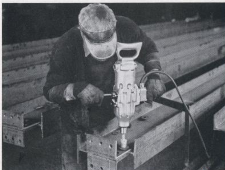
Locating flange plates on structural steel beams with No. 32 Positive Clutch Driver and socket wrench. ↑
