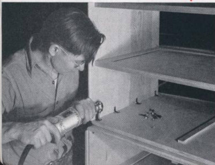
Furniture assembly. Driving Phillips Head screws with 90° Angle Drive Scrugun.
