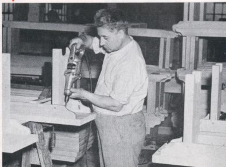
↓ Uniform tightness in furniture assembly is assured with No. 22 Adjustable Clutch Driver.
